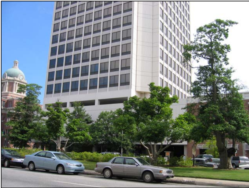
Front of Building
